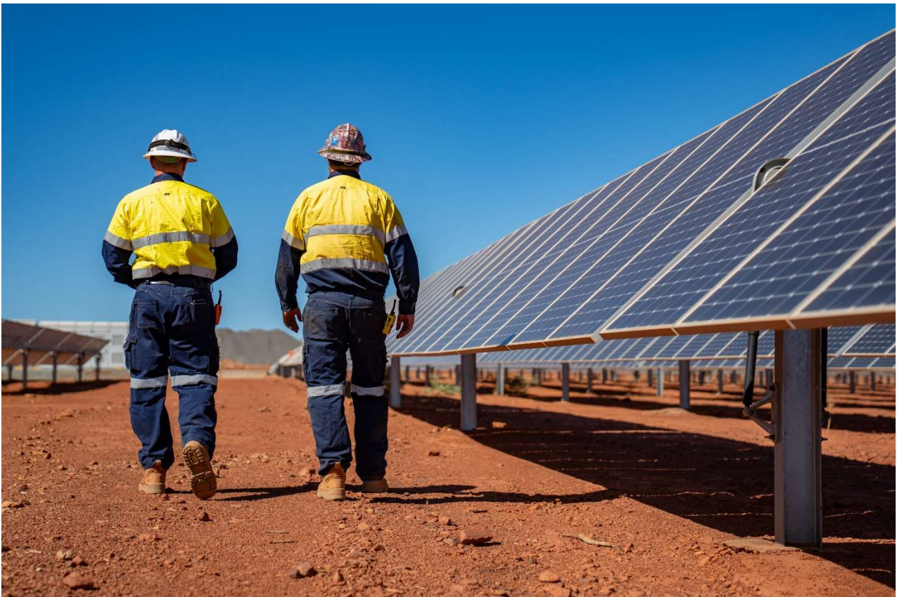
Figure 1 - Endurance employees inspect 11-hectare solar farm at Abra
